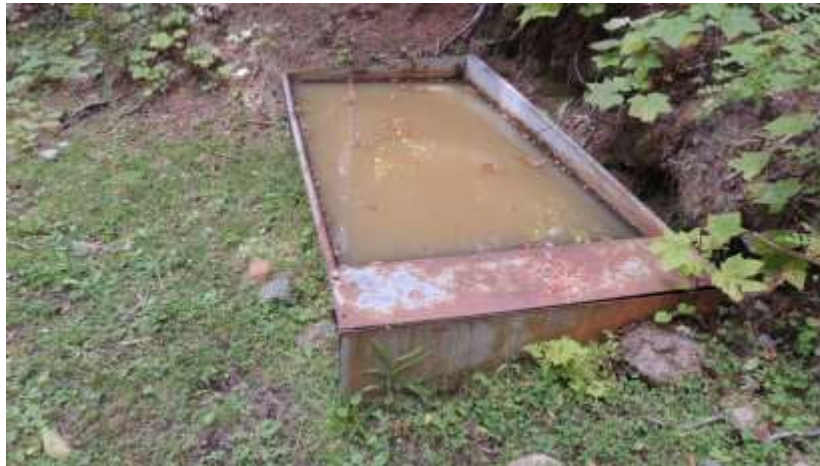
Figure 1 Stagnant, mosquito filled waterer as seen at Ingram & Johnstone Creeks. Cows avoid such water and go back to creeks.
