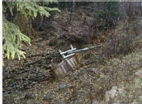
Fairly typical broken down cattle waterer that has not been maintained. Poor location in stream bed has resulted in washout.
